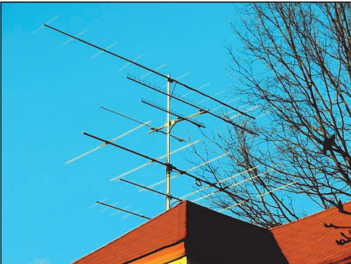
6 Foot fiberglass crossbar, with 3 loopers just below the top (2 Meter) antenna and above the 6 Meter antenna
